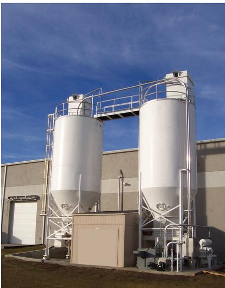
Condensation and high humidity can lead to product spoilage in bulk storage and cause blockages in pneumatic conveying applications.
